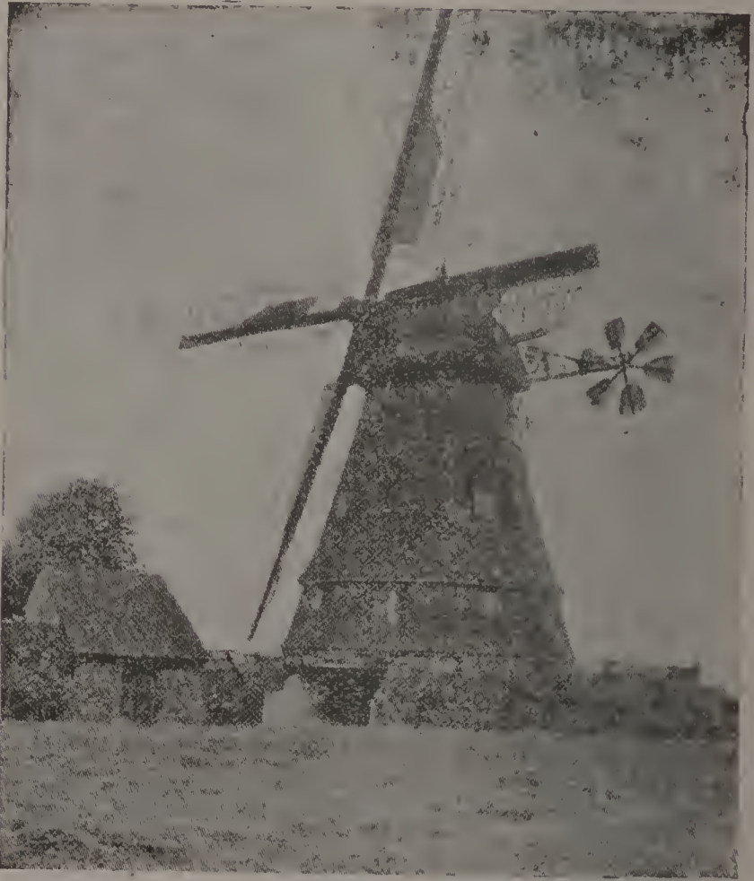
FIG. 3.—Tower Mill with Regulating or Wind Wheel.
